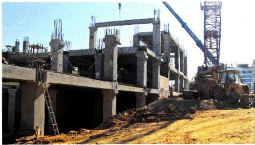
Precast technology has been adopted for faster execution and achieve quality construction with less wastage.
