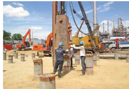
Concrete piling works
