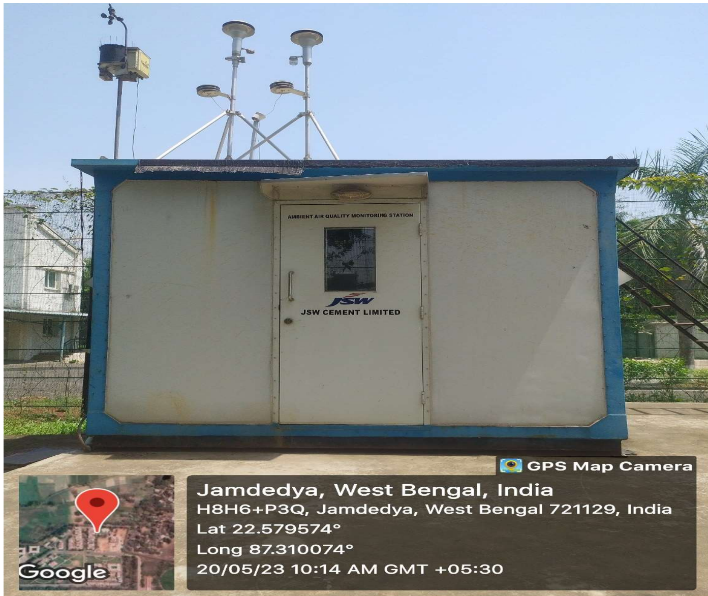
Continuous Ambient Air Monitoring Station (Photograph - III)
