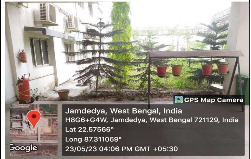
Fire Fighting System (Photograph-XXXIII)
