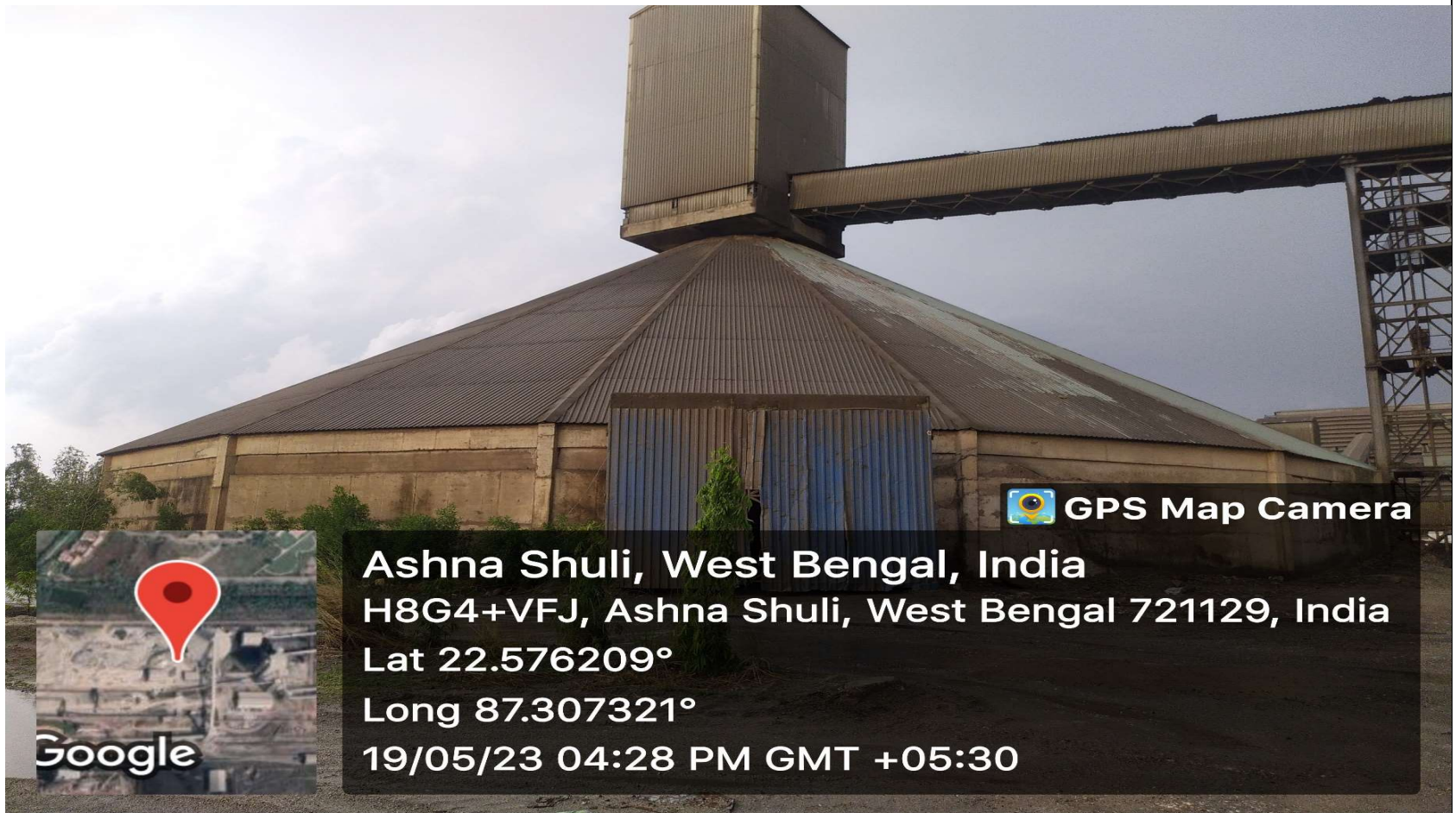
Closed Clinker storage RCC silo with APCD (Photograph - XV)
