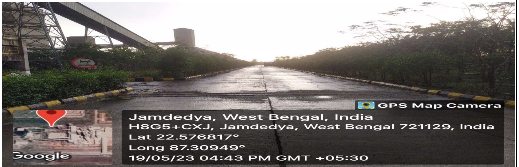
Plant inside Concrete road(Photograph - XXIII)
