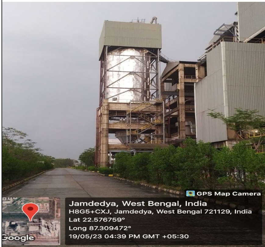
Covered Storage Bins (Photograph - VI)
