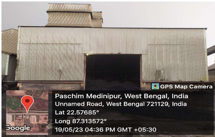
Covered RM Yard for Coal (Photograph - VIII)
