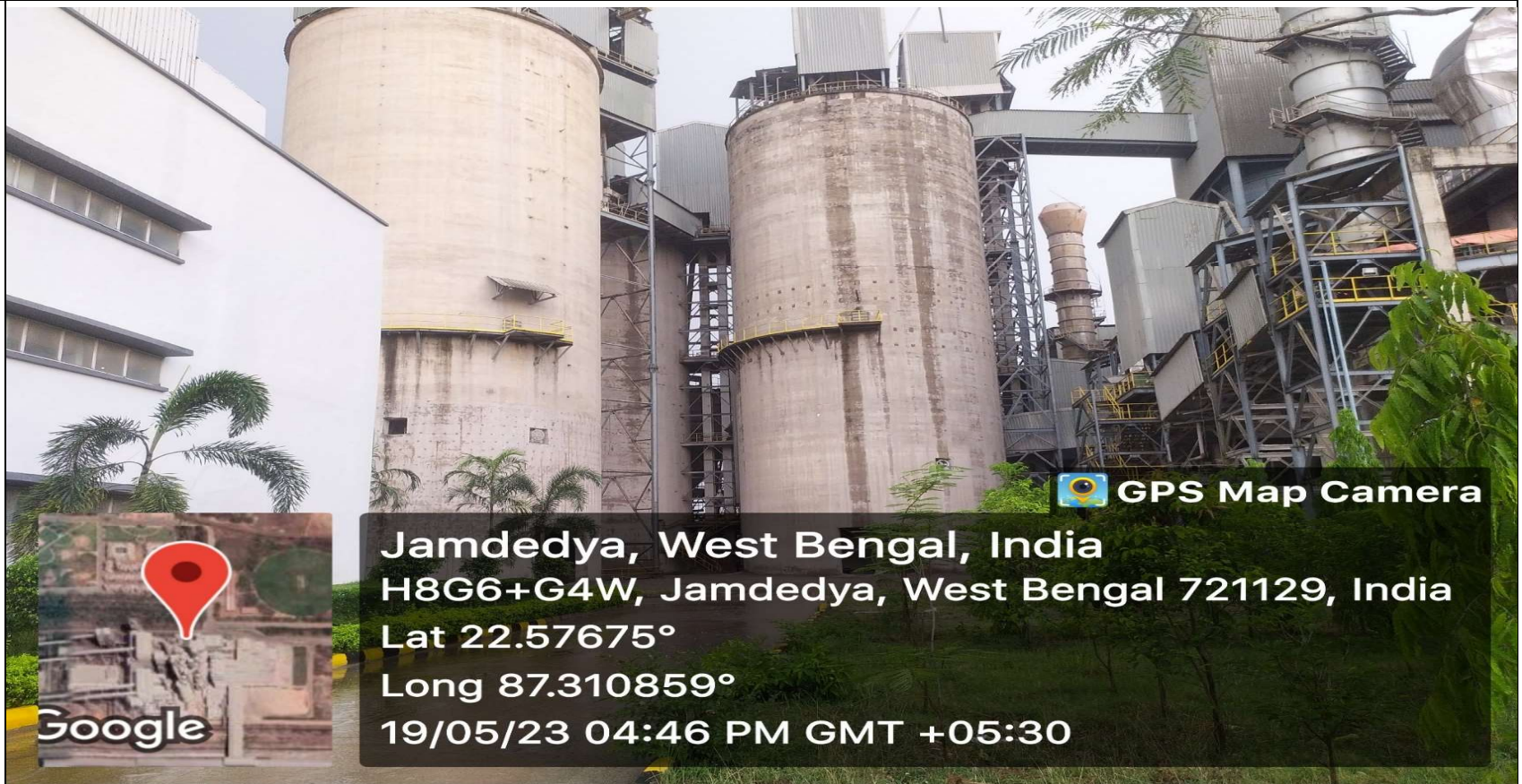
Closed Storage Silos with APCD(Photograph - IV)
