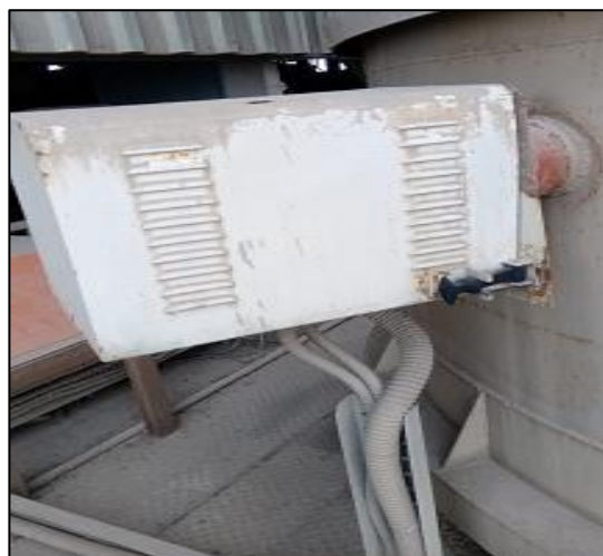
CEMS installed for Cement Mill
