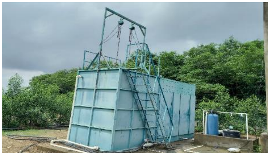
Fig 2. Water pollution Control Measure (STP of capacity 20 KLD)
