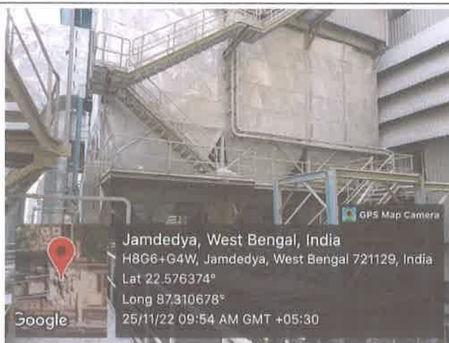
BAG HOUSE ATTACHED TO GRINDING UNIT : (Photograph-2)
