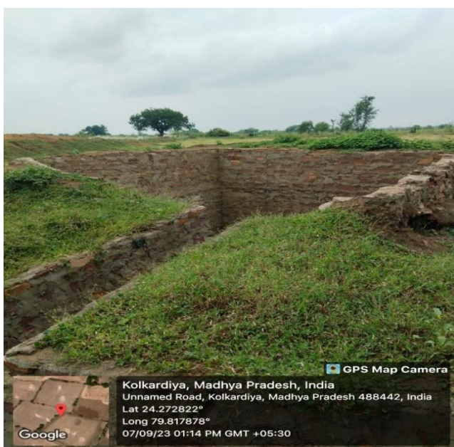
Siltation Pit -1 (L&W 5.3 and Depth 4.3 meter)
