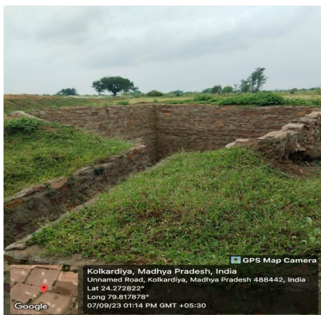
Siltation Pit -1 (L&W 5.3 and Depth 4.3 meter)
