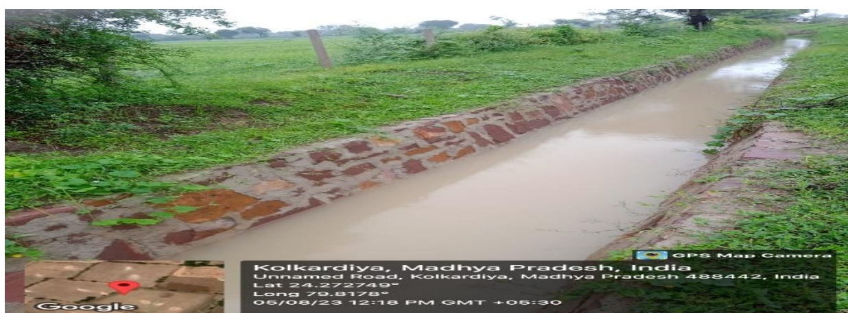
Rainwater Harvesting in Garland Drain
