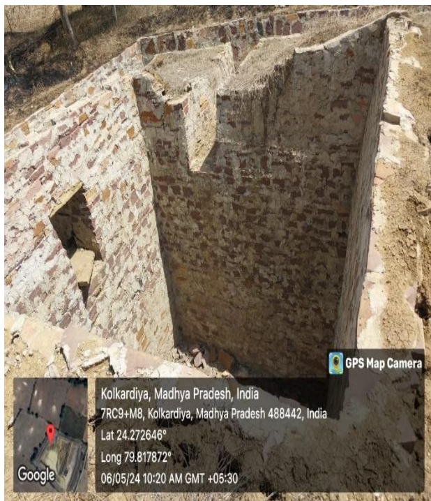
Siltation Pit -1 (L&W 5.3 and Depth 4.3 meter)
