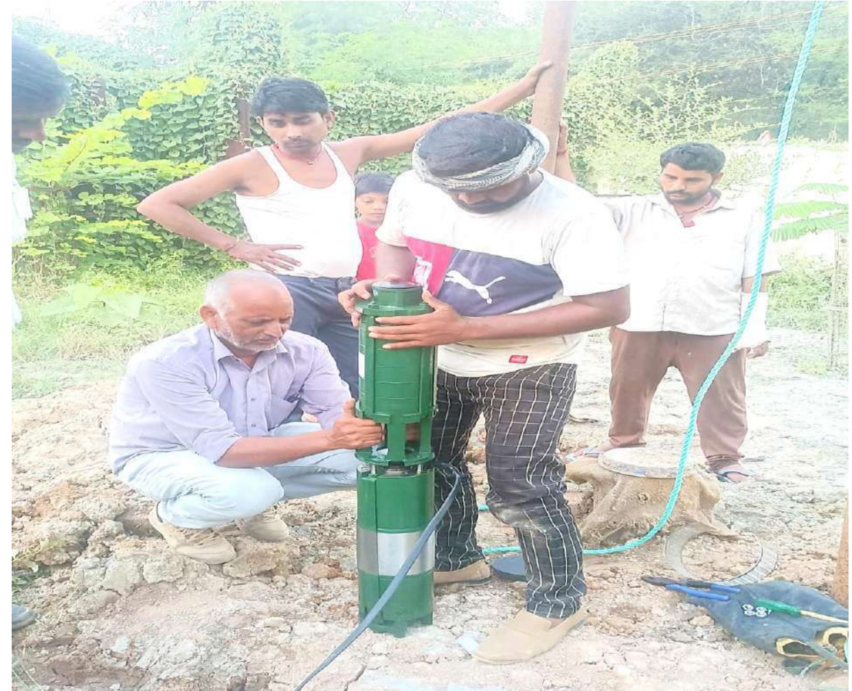
Photographs during fitting the Submersible pump at Kolkarhiya Middle School on 26 th Oct, 24
