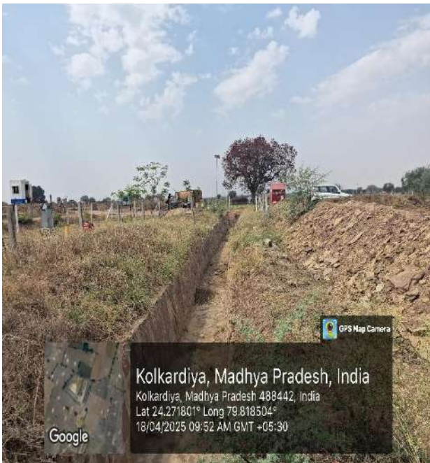
Photographs of the protected Garland drain by wire fencing along the pit area
