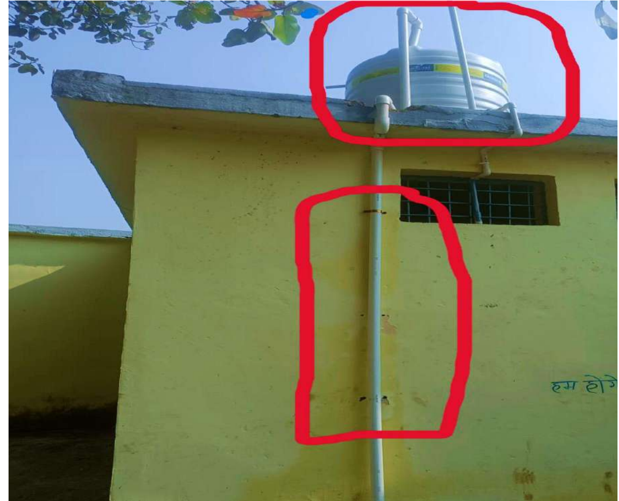
Water overhead tank connection fitting for continue water supply in School premises –Primary School on 22 nd Nov-2024
