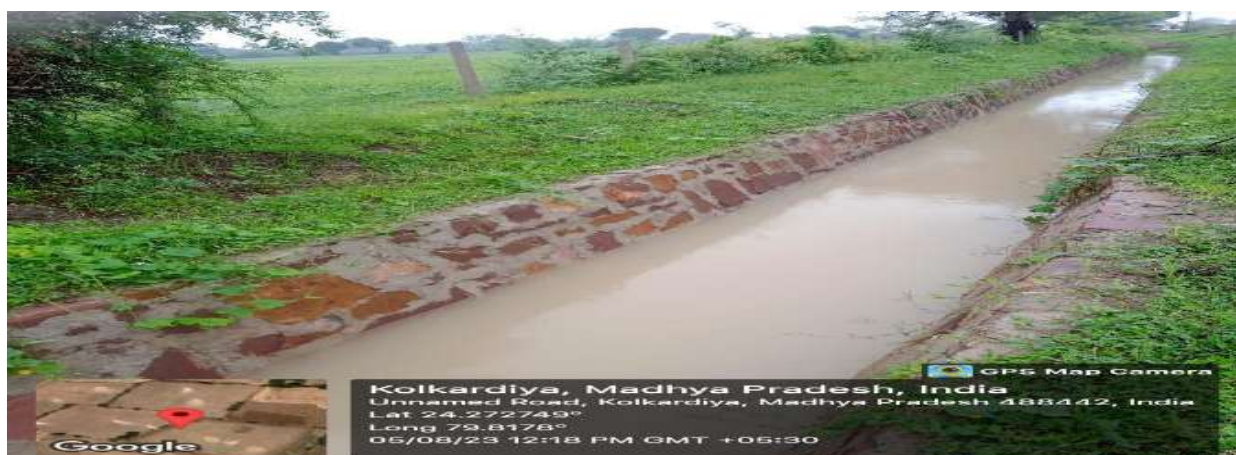
Rainwater Harvesting in Garland Drain
