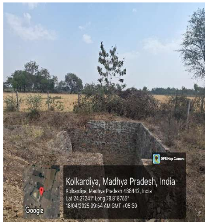
Siltation Pit -2 (L&W 5.5 and Depth 2.8 meter)
