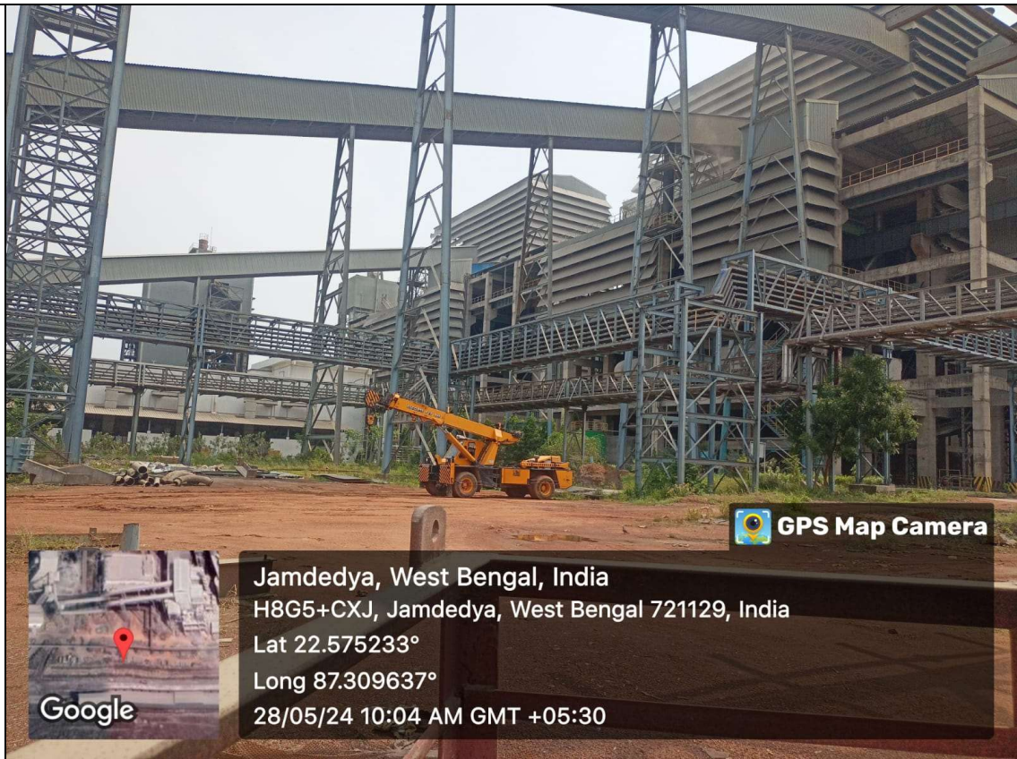
(Photograph-13) Enclosed Belt conveying System
