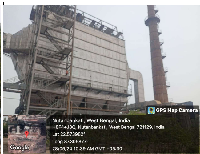
ESP ATTACHED TO CPP (Photograph-3)
