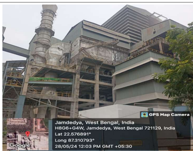
BAG HOUSE ATTACHED TO GRINDING UNIT : (Photograph-2)
