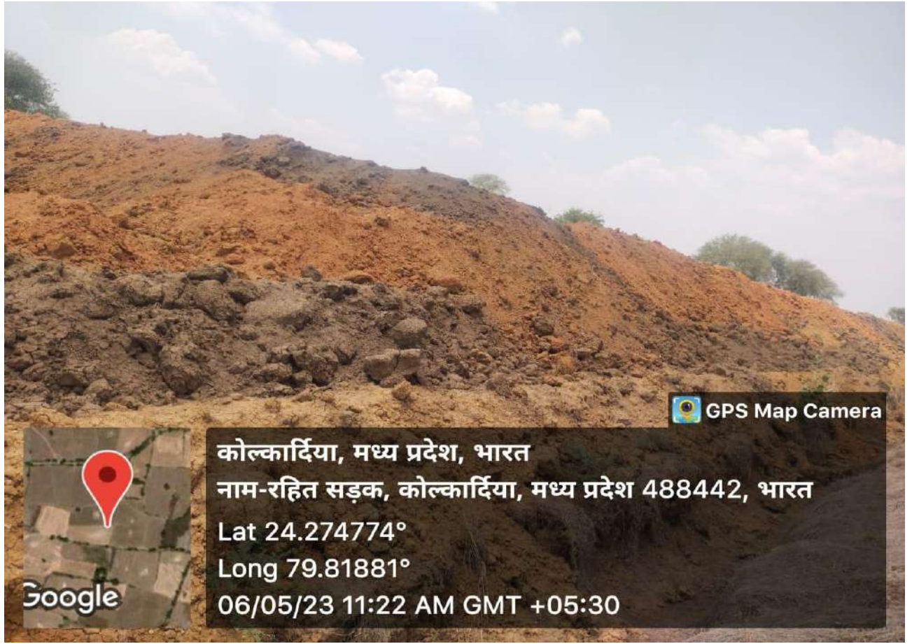
Photographs of bund under development along proposed excavation area
