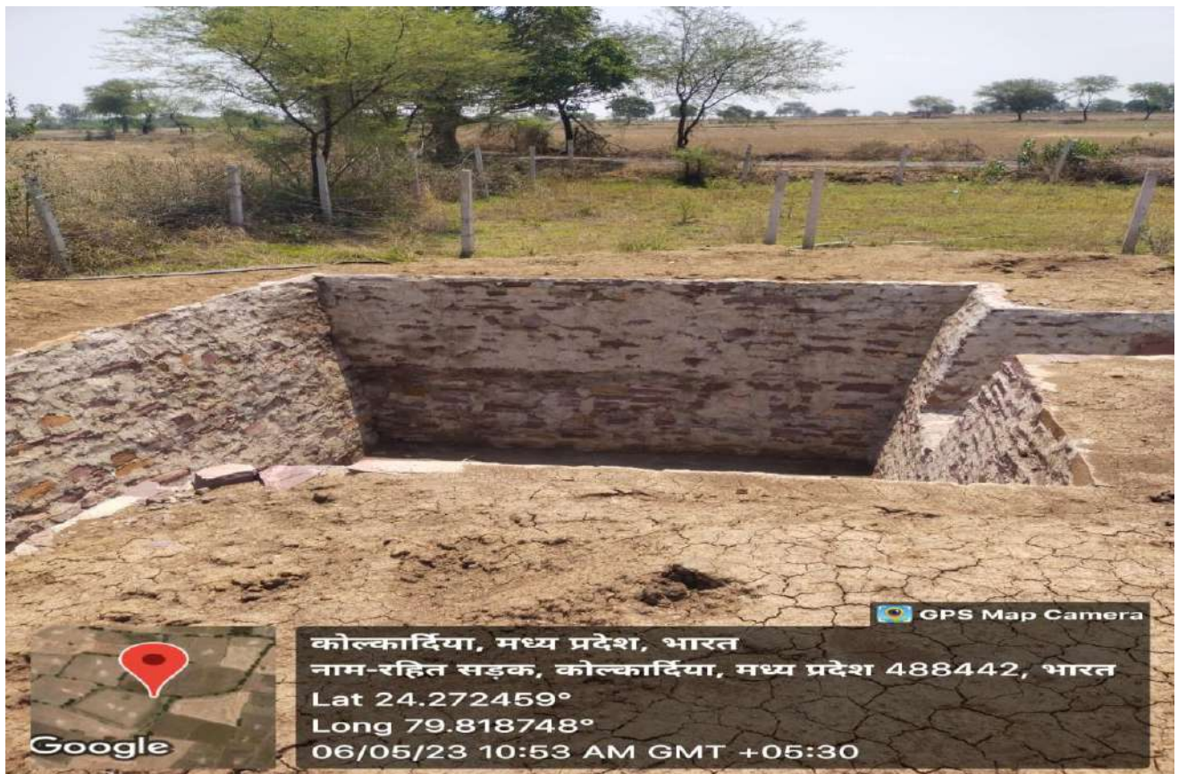
Photographs of protected Garland drain and siltation pond by wire fencing along pit area
