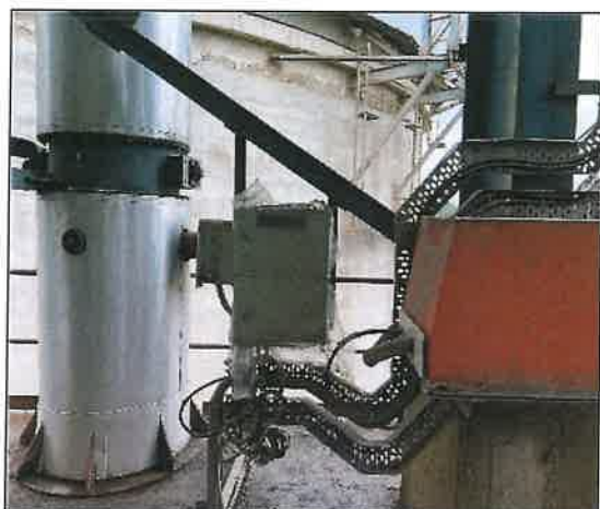
CEMS installed for Coal Mill
