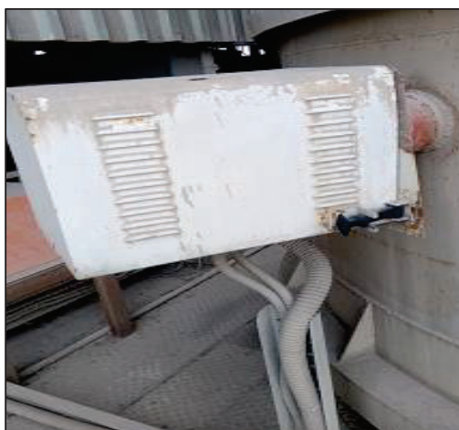
CEMS installed for Cement Mill
