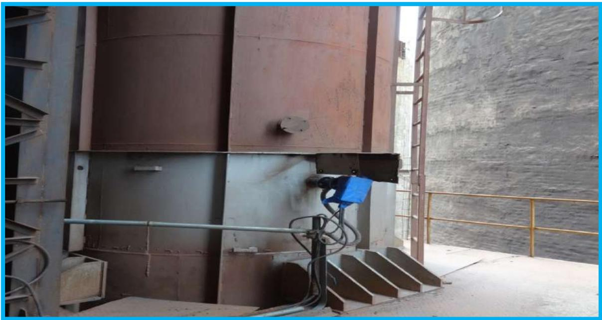
**CEMS Installed at VRM Bag house stack**
