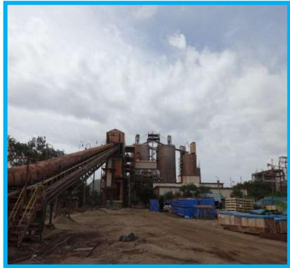
Bag filters provided at raw material transfer point with covered beld conveyer
