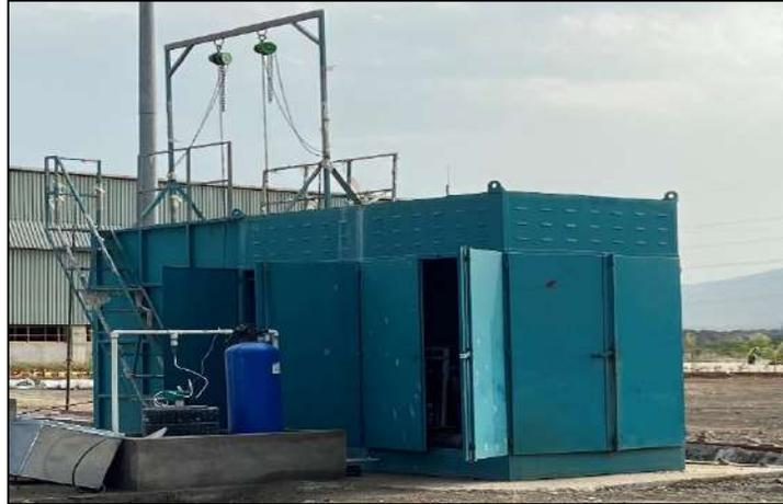
Fig 2. Water pollution Control Measure (STP of the capacity 20 KLD)
