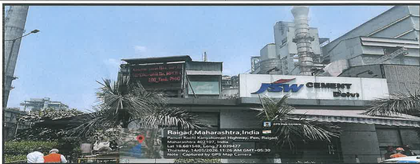
Photograph – 17: Online Display of environmental monitoring data at plant main gate
