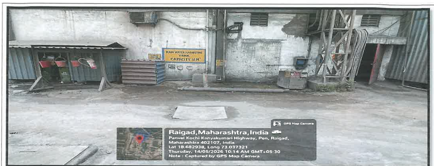
Photograph – 4: RWH Tank
