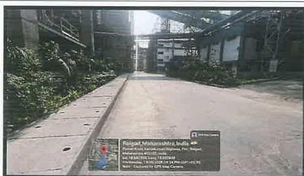
Photograph – 5: Covered storm water drain line
