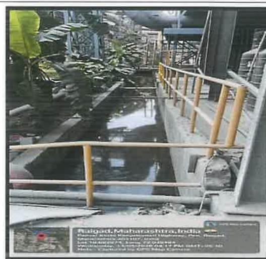
Photograph – 6: Desilted drain line
