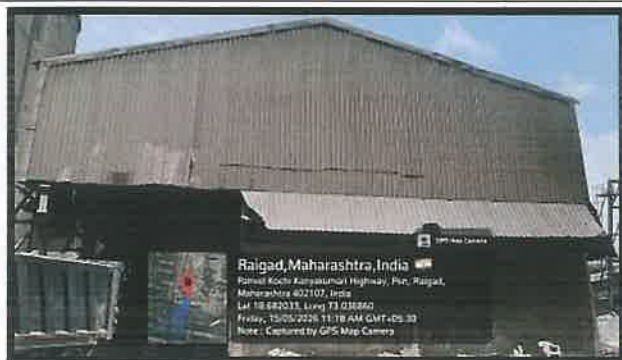
Photographs 8: Covered RM(Gypsum) Shed
