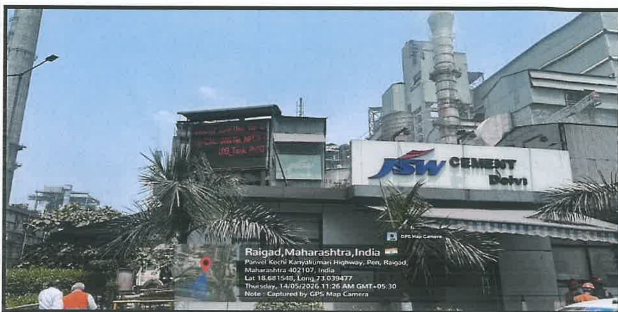
Photograph : 18 Environmental Display board
