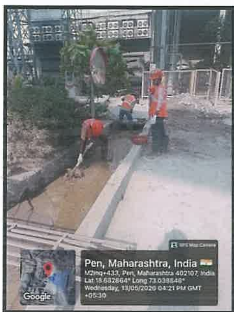
Photograph 15: Drain cleaning work
