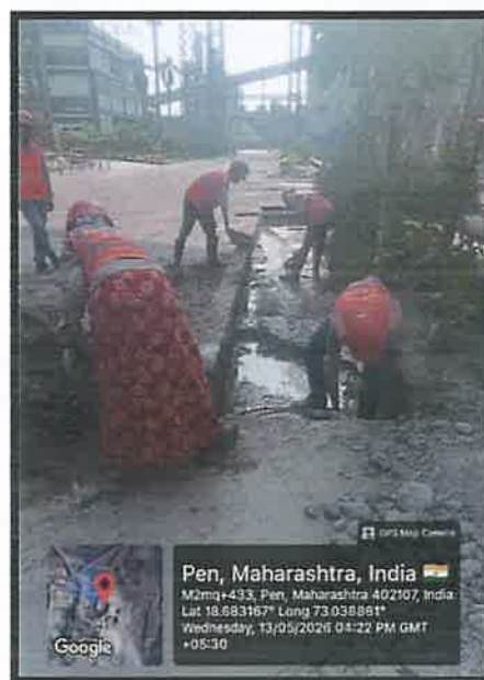
Photograph 16: Drain cleaning work
