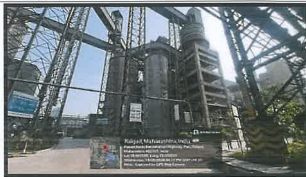
Photographs 7: Cement Silos
