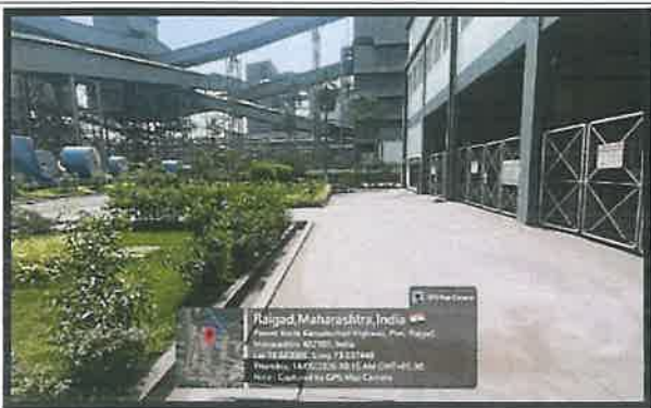
Photograph – 1 – Plantation near Admin Building
