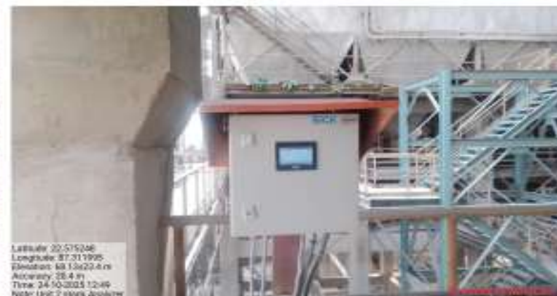
CEMS Analysers Attached with Cement Mill, Ball Mill & CPP
