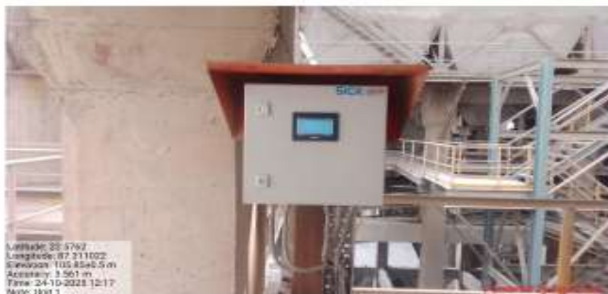
CEMS Analysers Attached with Cement Mill, Ball Mill & CPP
