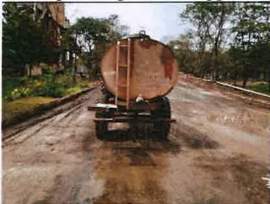
Water sprinkling for dust suppression (Annexure-7)
