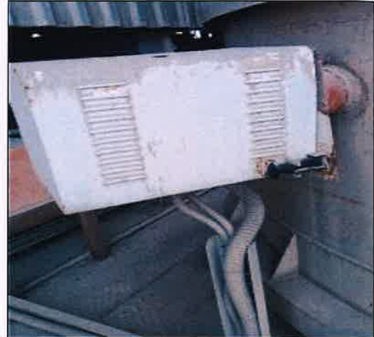
CEMS installed for Cement Mill
