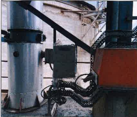
CEMS installed for Coal Mill
