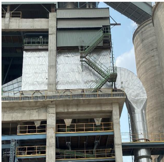
Main baghouse of the Roller Press
