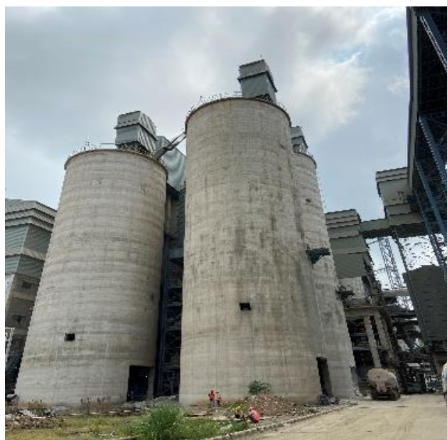
Closed Silo installed for Final Products
