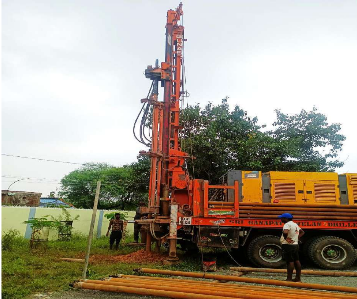
Photograph while Borewell digging at Kolkarhiya Middle School on 22 th Oct, 24
