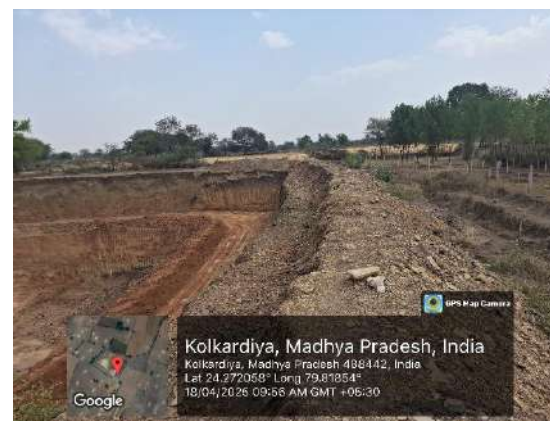
Bund along-with Mine Pit
