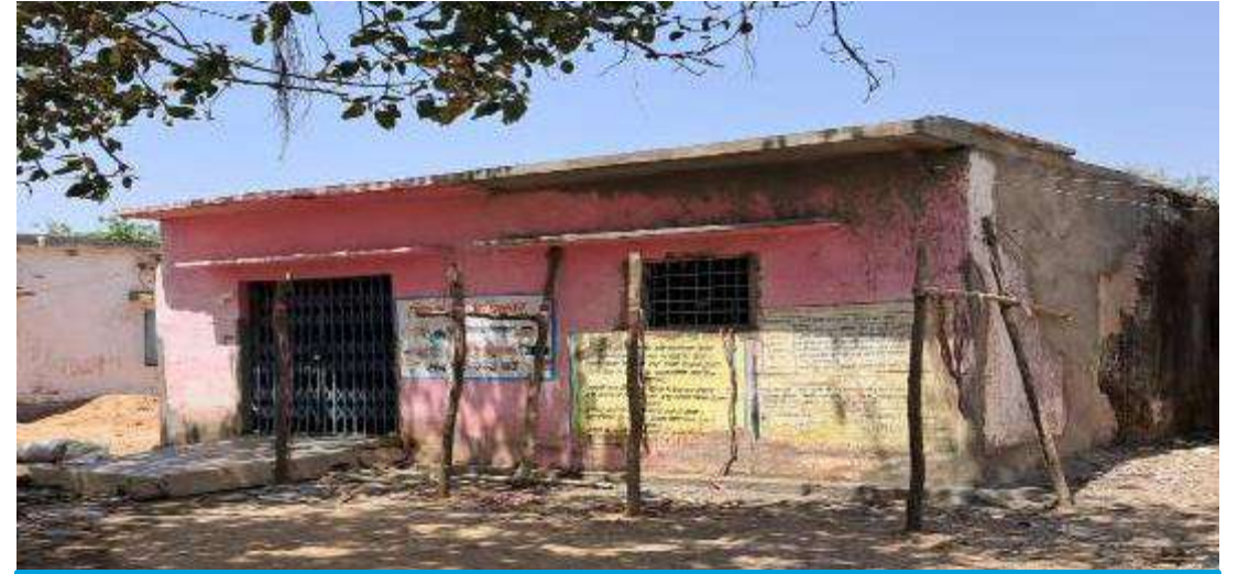
Primary section building before renovation
