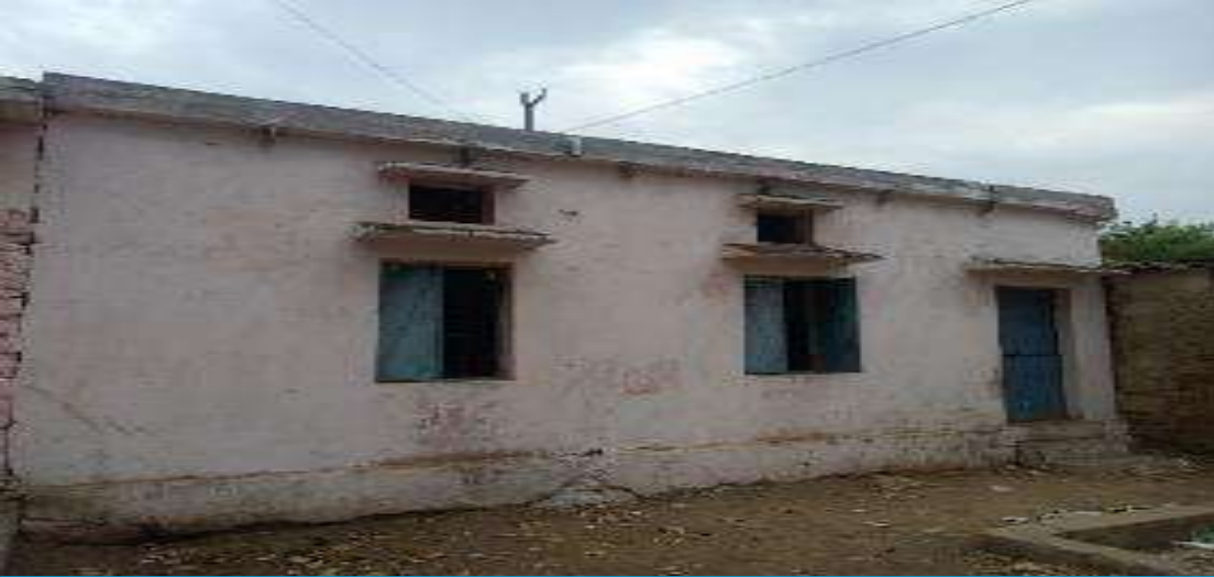
Primary and Kitchen section building before renovation
