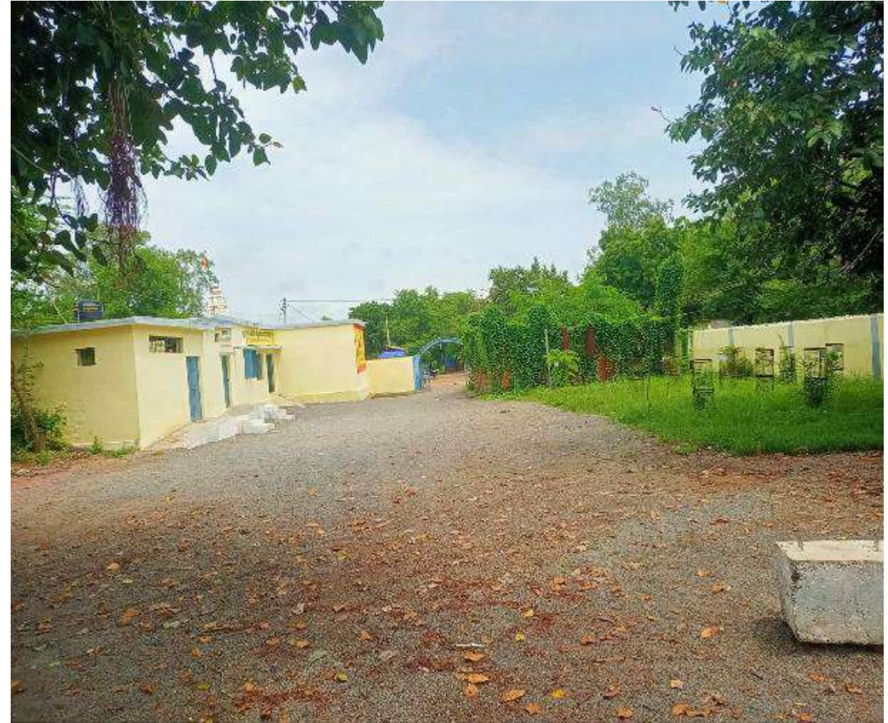
Ground development and boundary wall renovation
