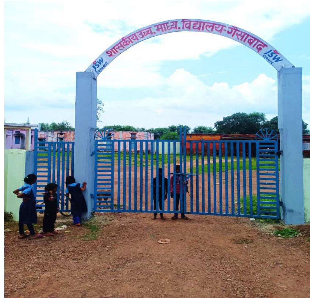
Higher Secondary School Main Gate Section after renovation
