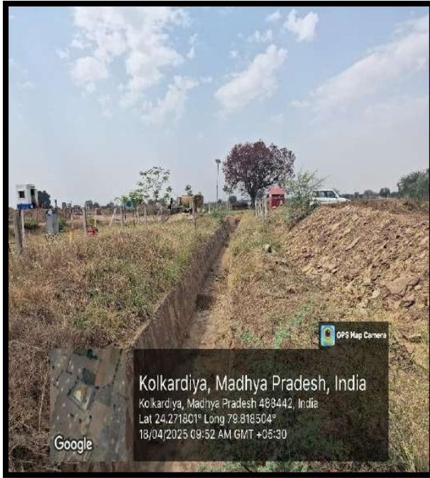
Photographs of the protected Garland drain by wire fencing along the pit area
