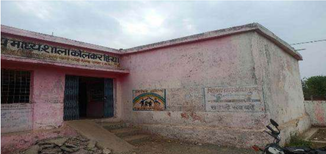
Middle section building before renovation
