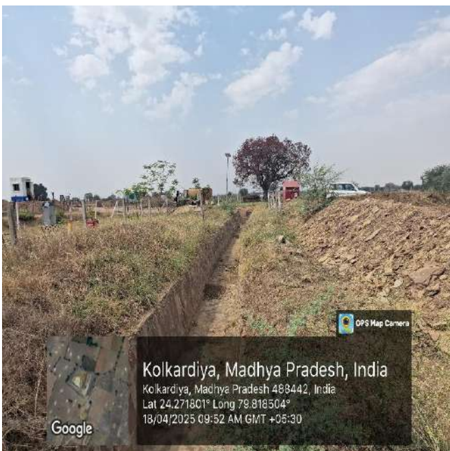
Photographs of the protected Garland drain by wire fencing along the pit area
