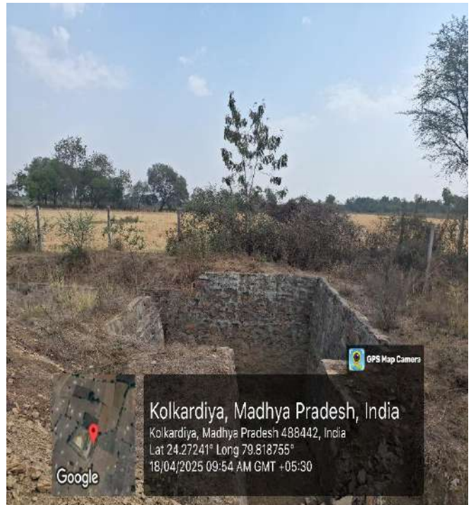
Siltation Pit -2 (L&W 5.5 and Depth 2.8 meter)
