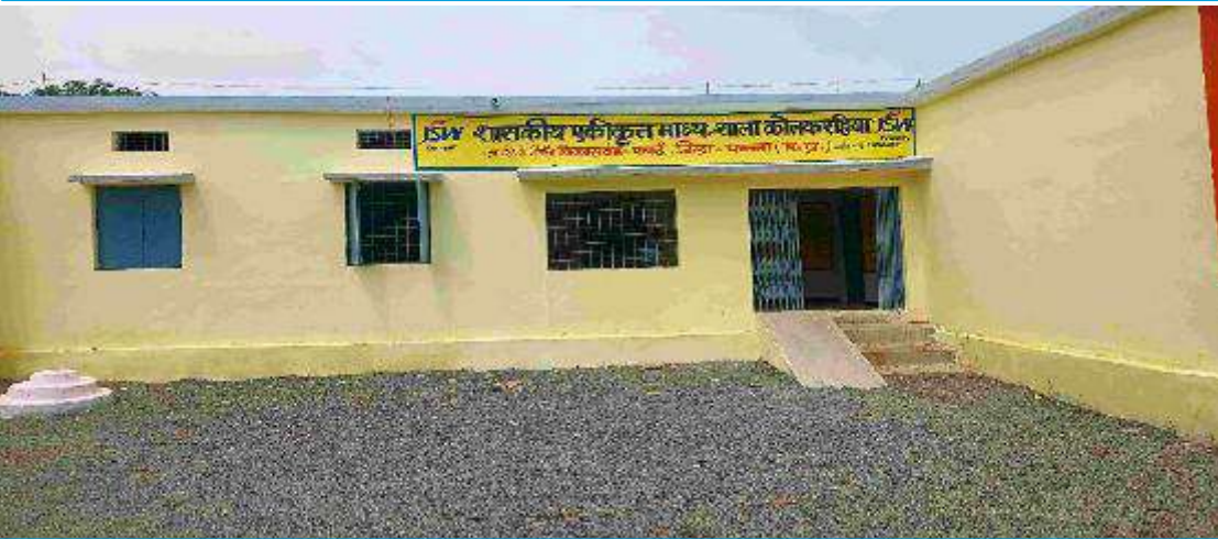
Middle section building after renovation
