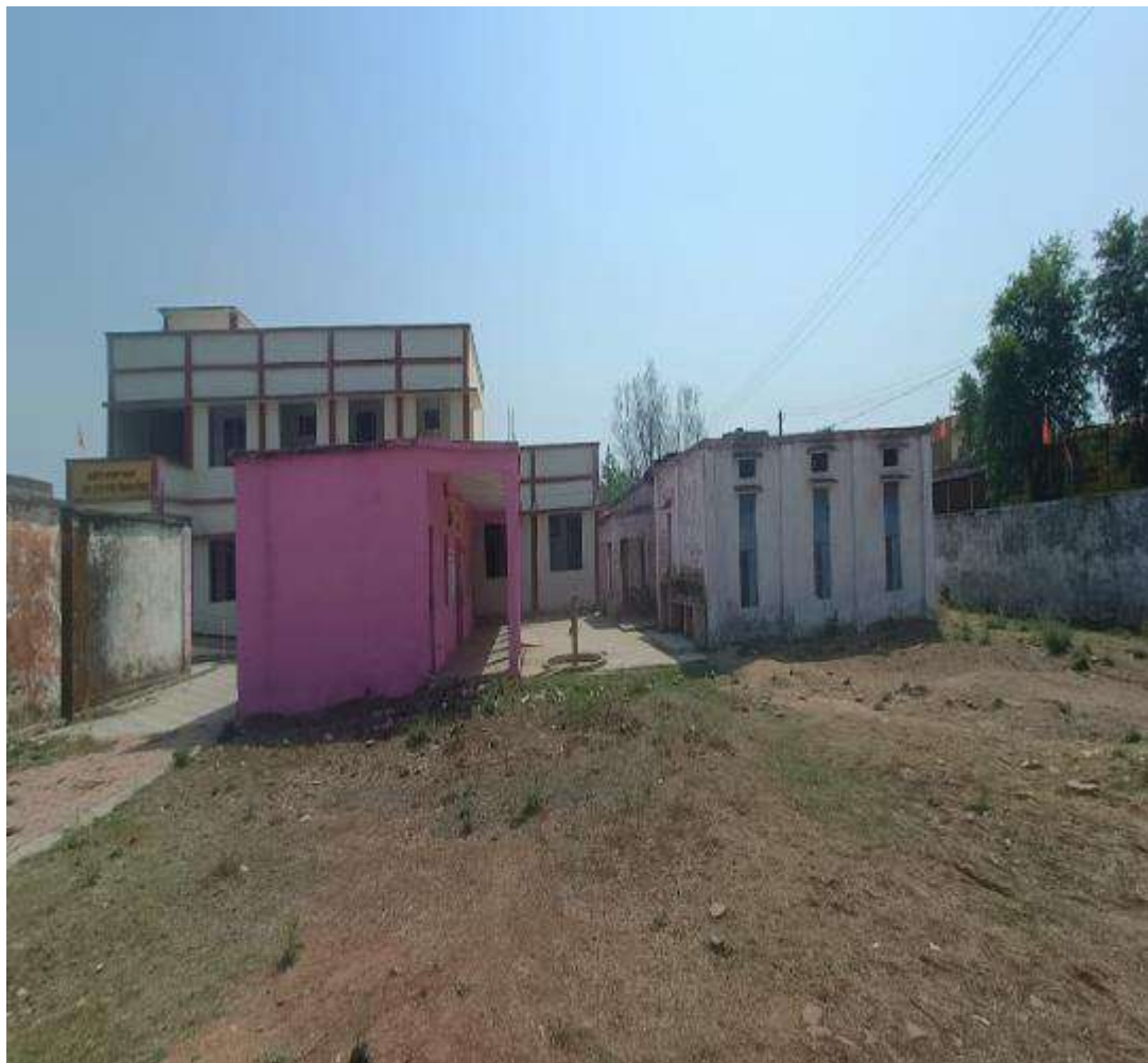
Primary School Section before renovation & Cycle stand
