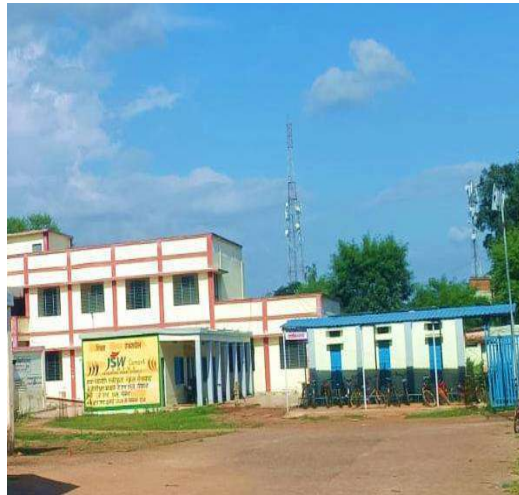
Primary School Section after renovation & Cycle stand
