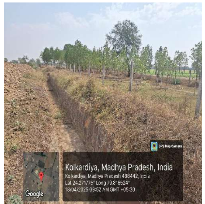
Photographs of the protected Garland drain by wire fencing along the pit area
