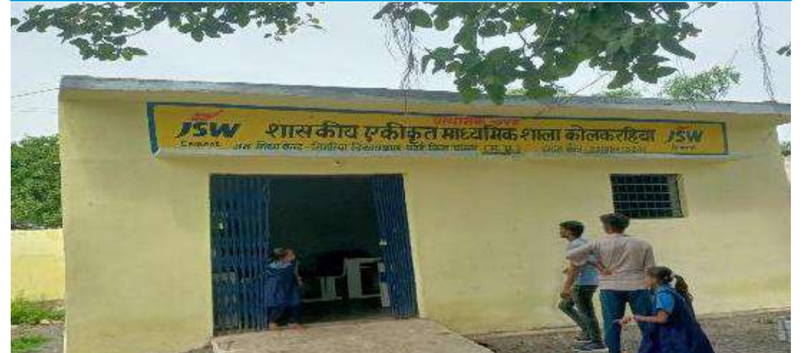
Primary section building after renovation
