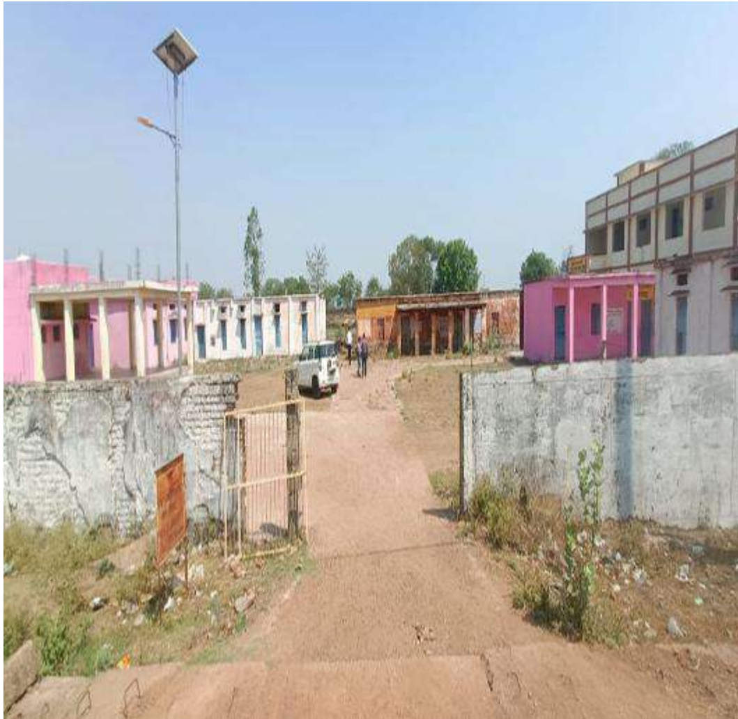
Higher Secondary School Main Gate Section before renovation
