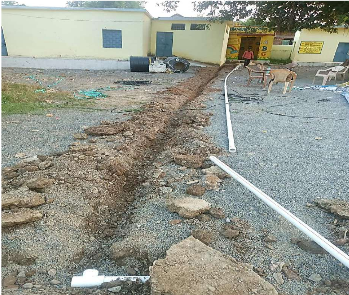
Photographs during fitting the pipeline on 11 th Nov, 2024
