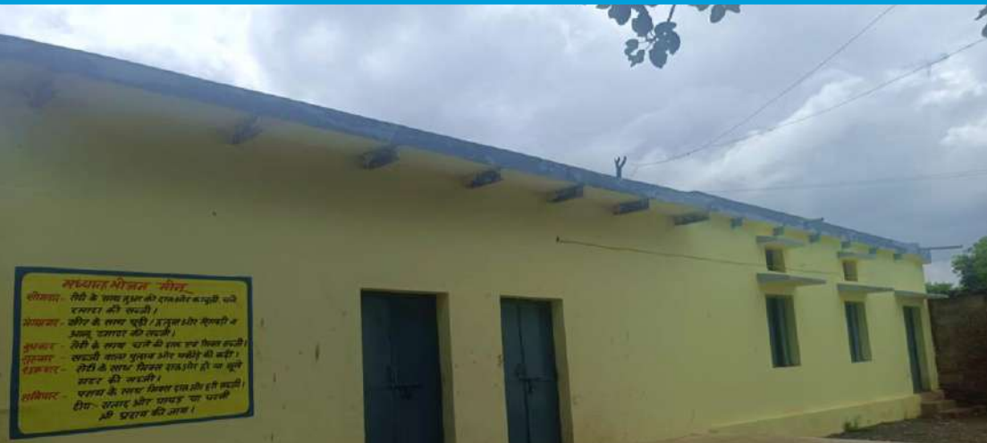
Primary and Kitchen section building after renovation
