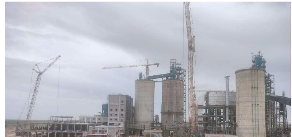
Nagaur IU – cement grinding, packing & dispatch
