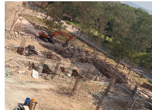
Baghouse and MCC Room
