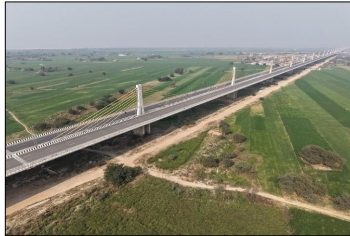
L&T Daewoo- Patna Bridge
