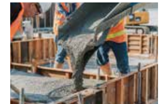
Foundations and retaining walls
