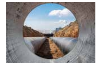
Water-retaining and sewage structures
