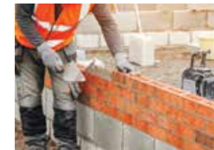
Brick masonry and plastering
