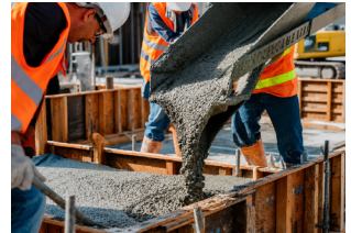
Foundations and retaining walls
