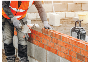
Brick masonry and plastering
