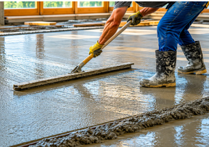
RCC works requiring quick setting and early strength
