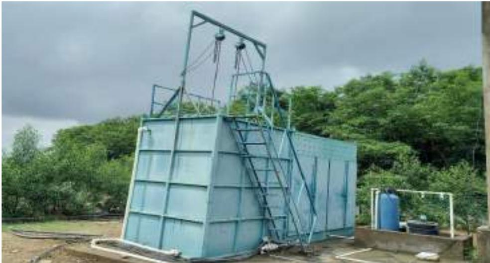
**20 KLD Sewage Treatment Plant installed for treatment of domestic water**
