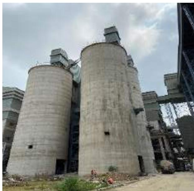
**Closed Silo installed for Final Products**
