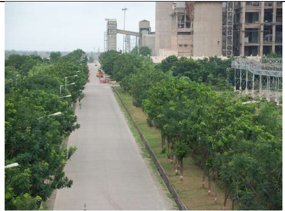
Description: Plant Internal CC Roads
