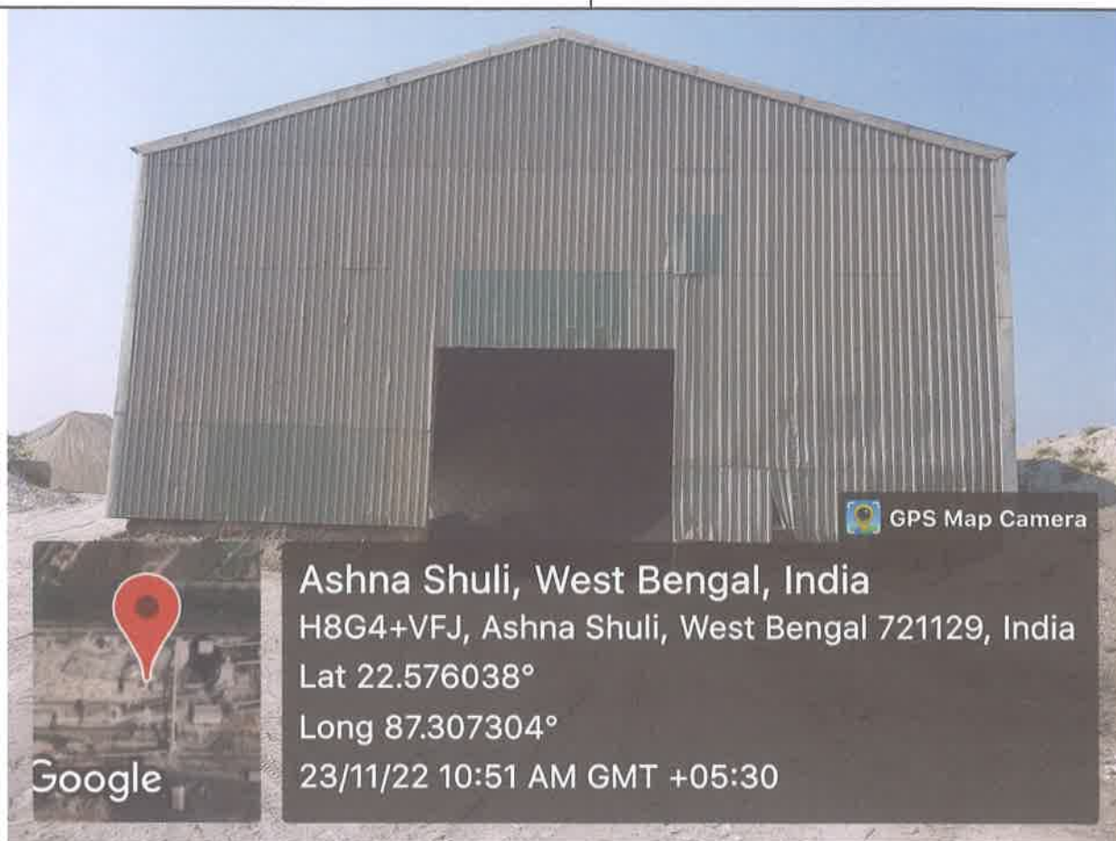
GYPSUM SHED Photograph no.-20
