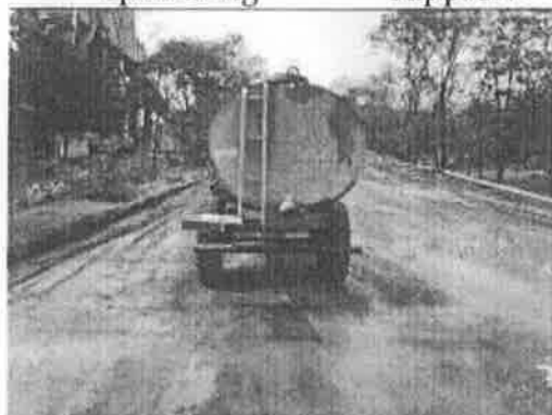
Water sprinkling for dust suppression (Annexure-7)
