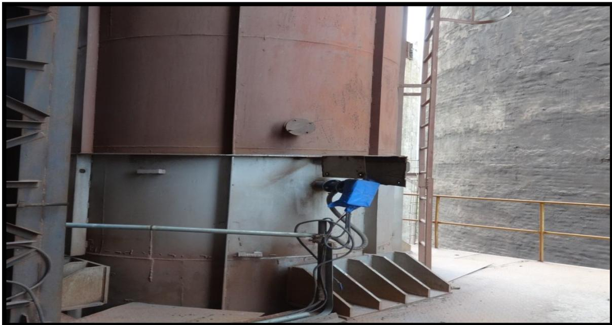
**CEMS Installed at Cement mill stack**
