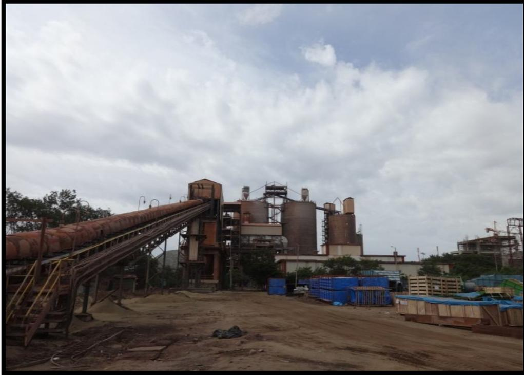
**Covered belt conveyer, silo with bag filter for the storage of cement & GGBS**
