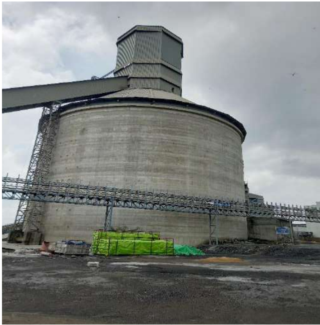
Clinker Storage Silo
