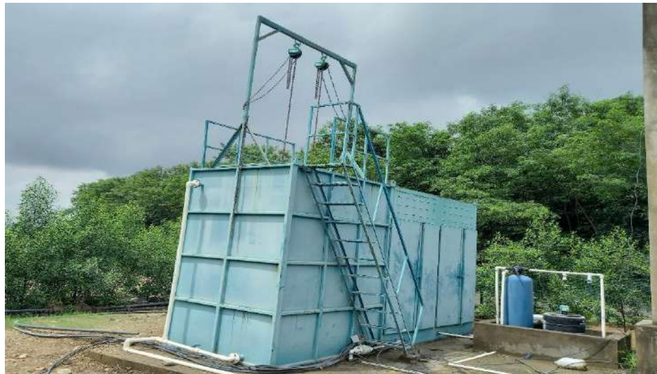
Fig 2. Water pollution Control Measure (STP of the capacity 20 KLD)
