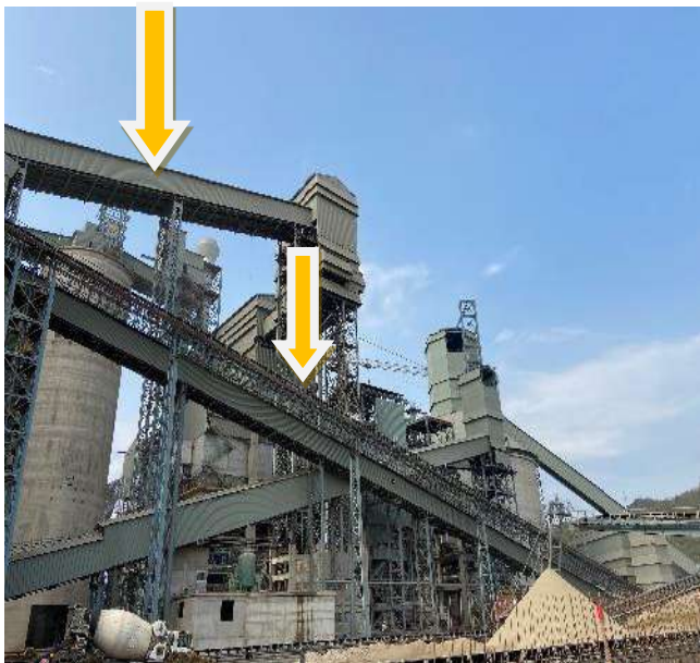
Closed conveyor belt with bag filters at all transfer points
