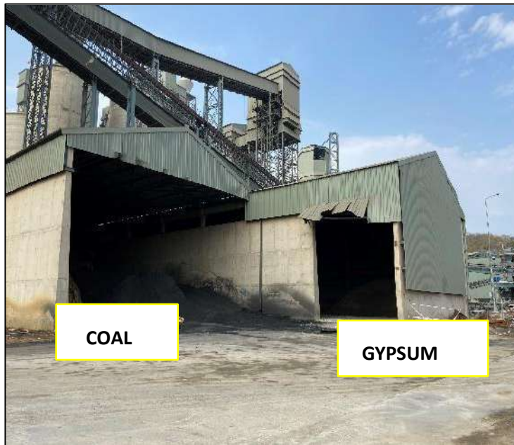
Coal and Gypsum Storage Yard
